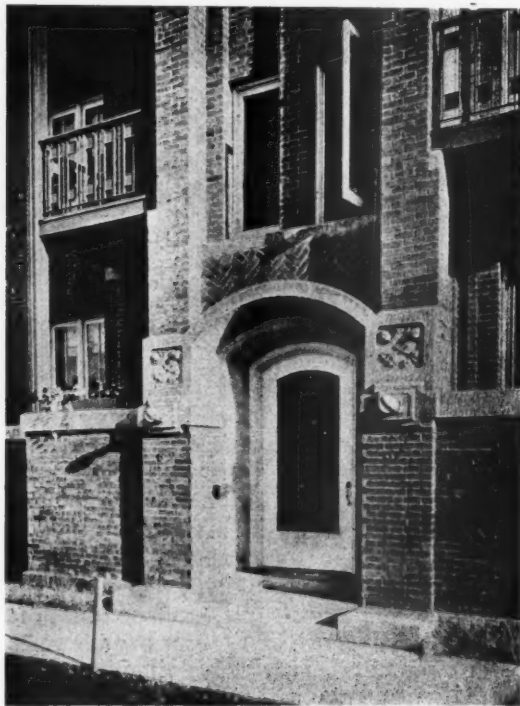
ENTRANCE DETAIL, APARTMENT HOUSE, CHICAGO, ILL.
